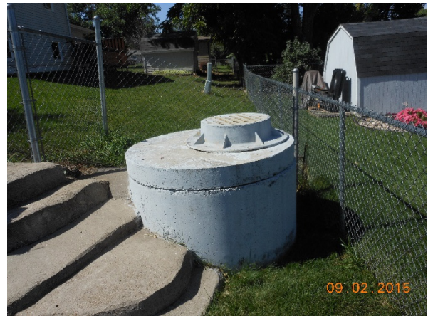
Photo 12. Storm Manhole North of Cedar Drive
