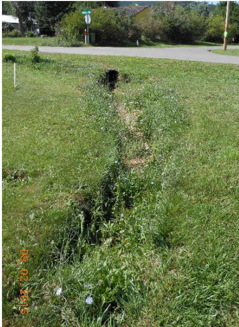
Photo 1. Area Discharge Outlet East Side of Vanocker Road and 1 st Avenue
